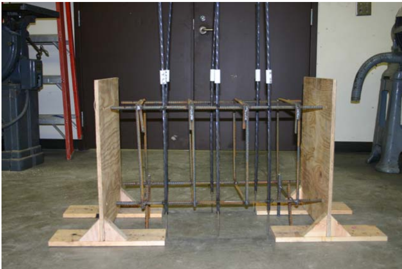
Figure 5-4 Wood Jig Used to Construct Cage for LBPT
