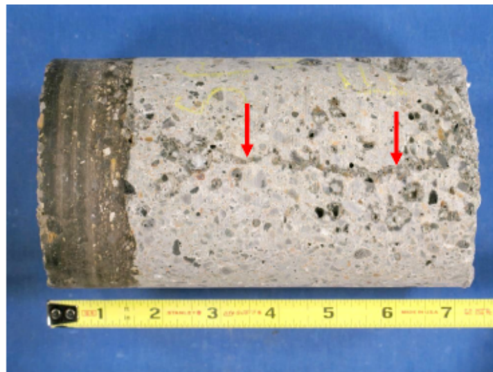
3b. Side view. Arrows indicate a vertical crack in the concrete. The photo was taken while drying after being wetted with water to highlight the crack. Top surface is to left.
