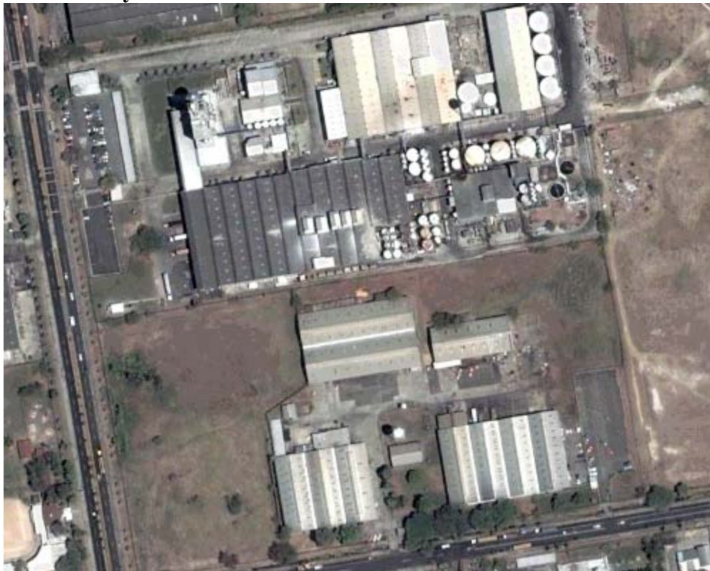
Figure 1.1 Factory Aerial View
