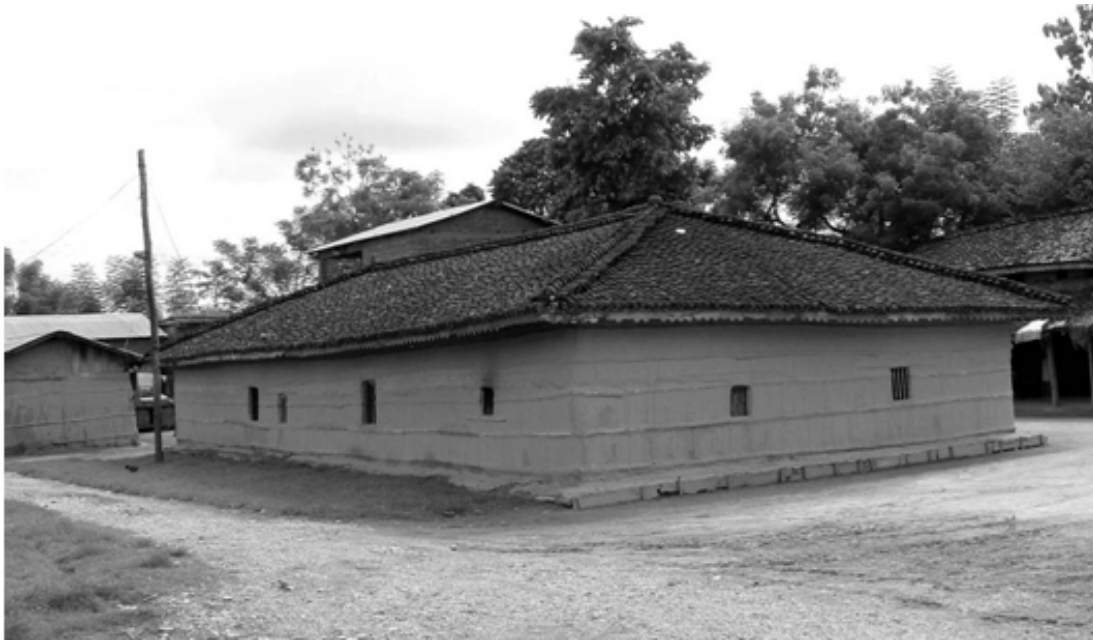
Figure 9. Author's photograph of a Tharu house showing small fenestrations, horizontal members of wattle and daub wall, and roof form, July, 2010.
