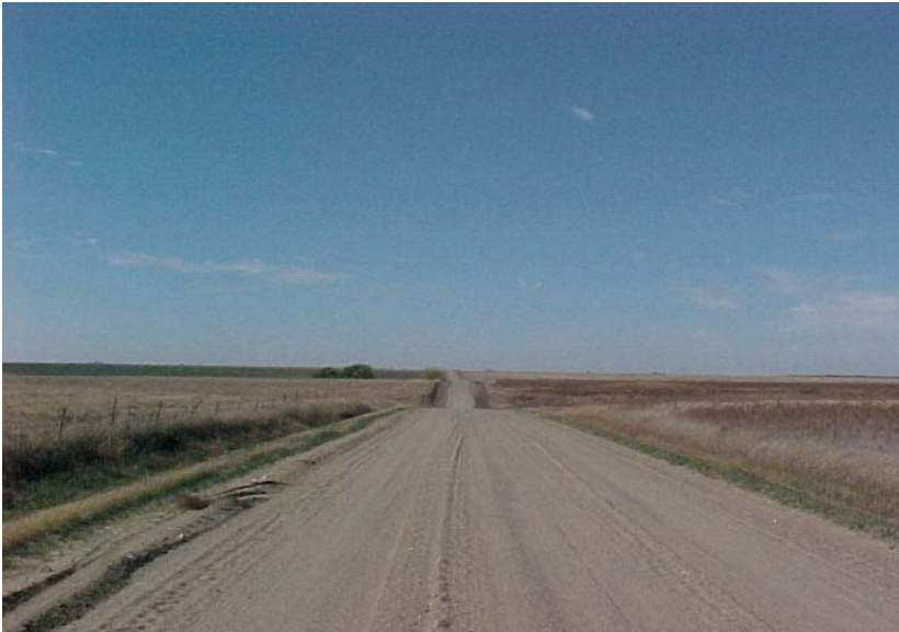
Figure 3.9 Golf Course Rd. in Trego County, Kansas
