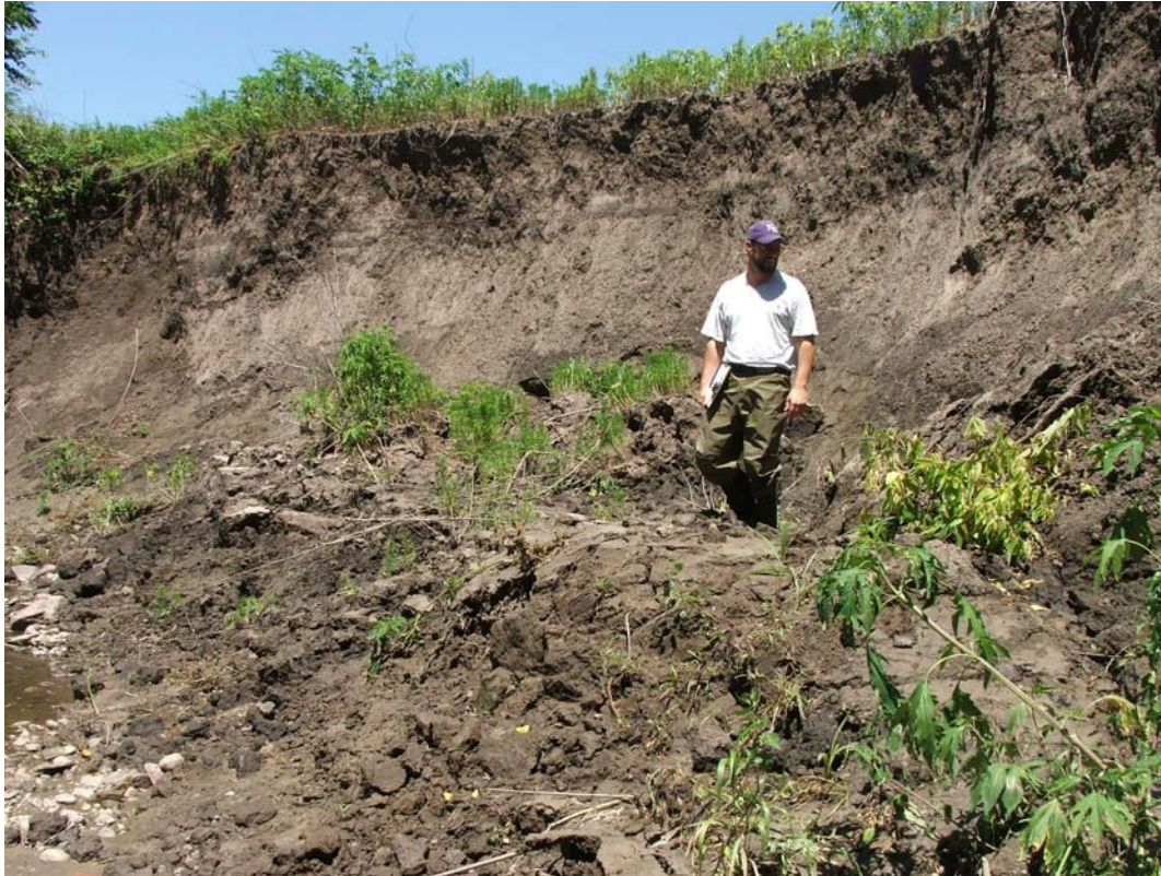
Figure 5.2 Irish Creek 2 study bank after June 2010 rains (Keane, 2010). Four-foot erosion pins were lost and the bank profile toe pin was buried.
