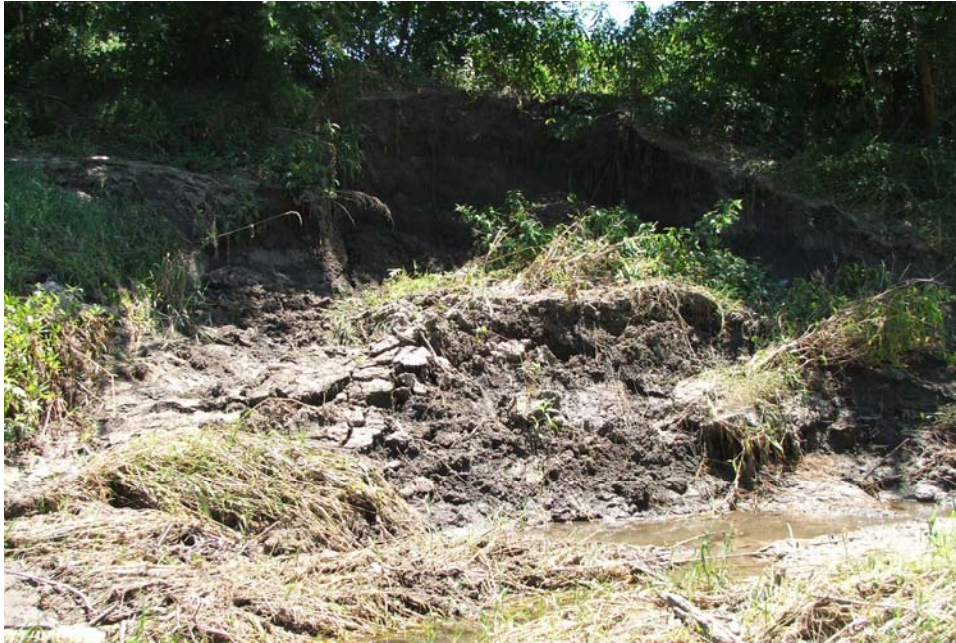
Figure 5.6 North Fork study reach 3 typical bank failure along reach establishing a new bankfull bench along both sides and re-vegetating streambanks (Keane, 2010).
