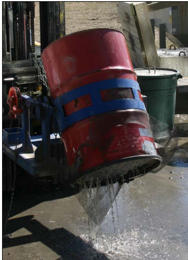
Figure 5.2. Water being strained from lightweight aggregate for large concrete batch.
