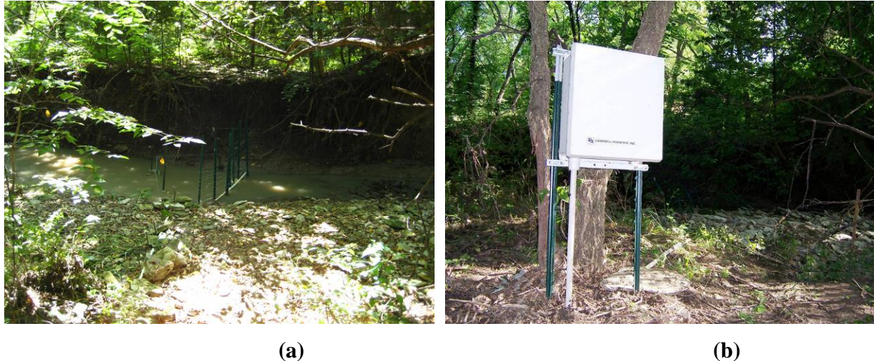
Figure 3.6 Little Kitten Creek site installation: a) Protection PVC pipe running from the creek to bank; b) waterproof enclosure that contains datalogger and the signal conditioning box.
