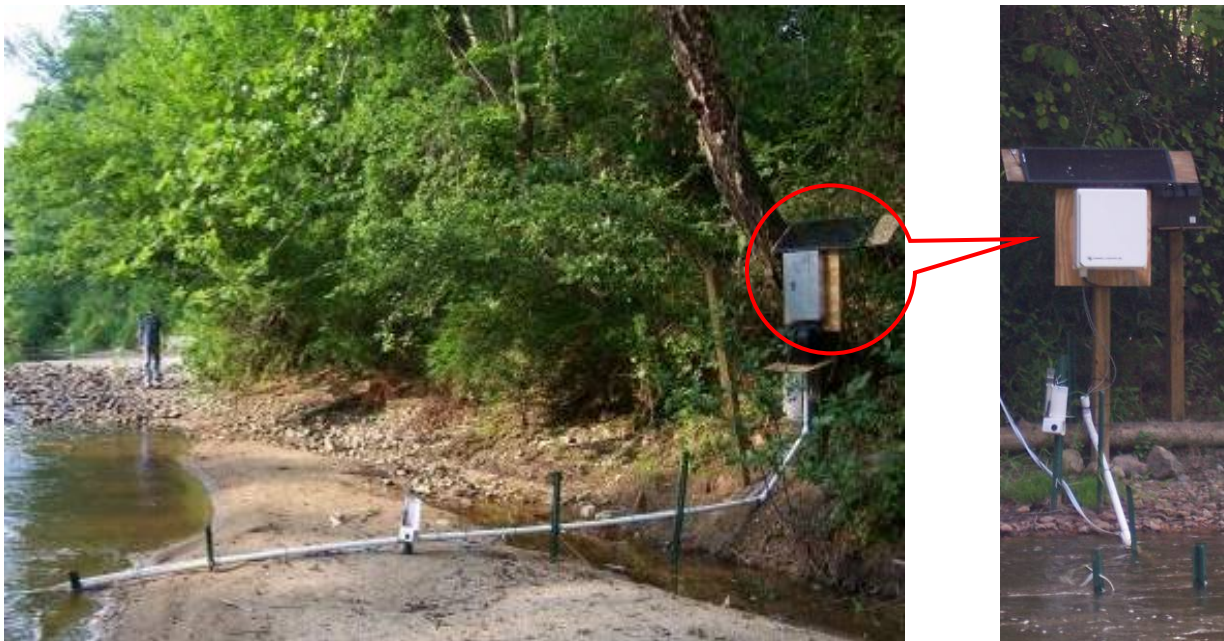
Figure 3.7 SSC measurement system installation at a LWSC in Fort Benning, Georgia.
