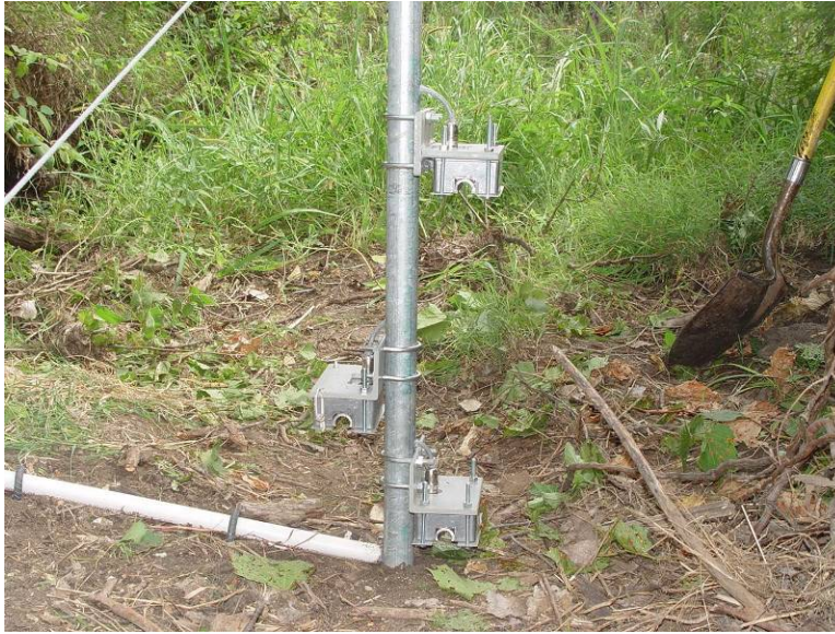
Figure 3.2 Sensors were mounting using a galvanized steel pipe at Fort Riley, Kansas.
