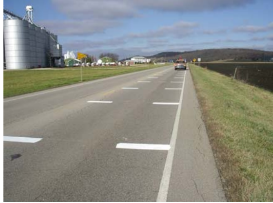
b. Optical Speed Bars on US-24/ US-59
