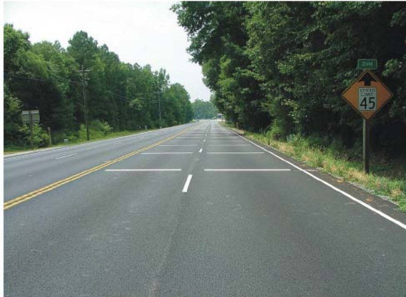
Figure 2.3 Optical Speed Bars on Route 460, East Side of Zuni
