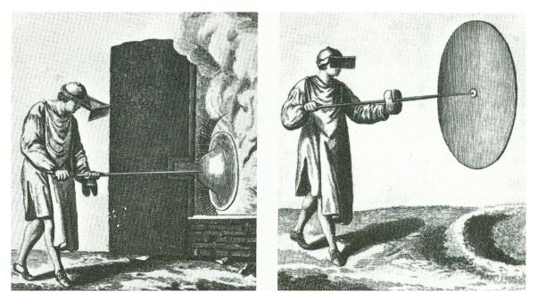
Figure 2-2 Method for Spinning Flat Glass (Maloney 63)
