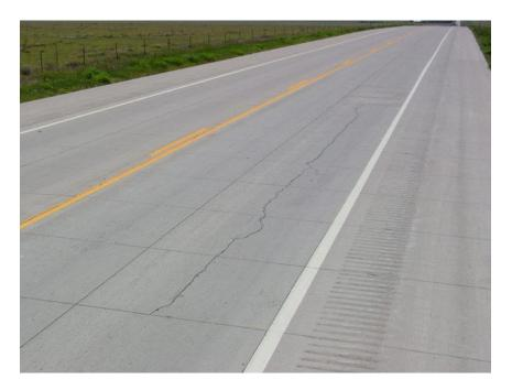
Figure 2.15 Typical Cracked Slab Conditions Observed at the U.S. 287 Lamar Site
