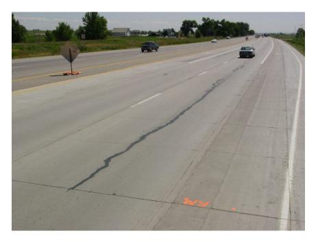
Figure 2.13 Typical Slab Cracking Observed in S.H. 119 Test Section No. 2 (Sheehan
