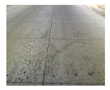
Figure 2.17 Hairline Crack in Kalispell Project Pavement (MtDOT, 2008)
