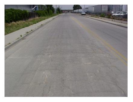
Figure 2.11 Stop Sign Approach Distressed Area Observed at Santa Fe Drive Site
