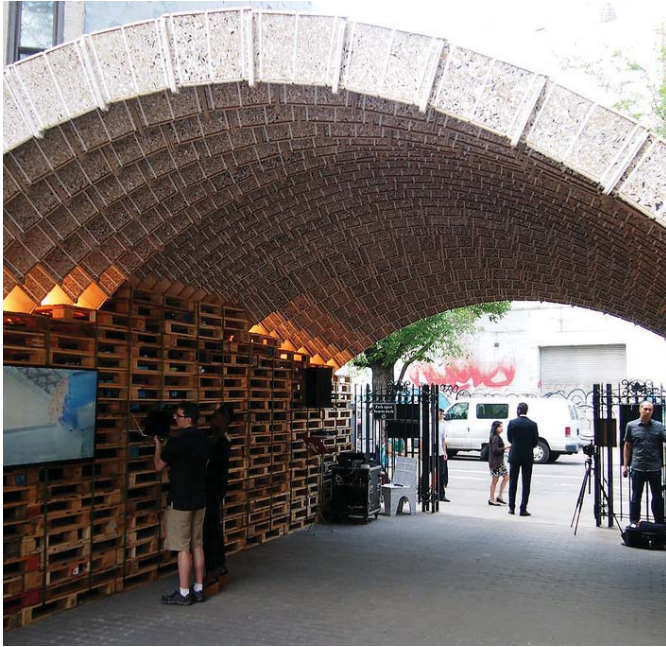
Figure 4.4 The ETH Zurich Future Pavilion (Les Architectures 2015)
