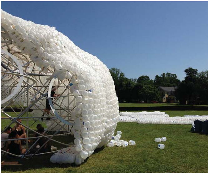
Figure 4.14 Construction of the Pavilion (Sheridan 2013)
