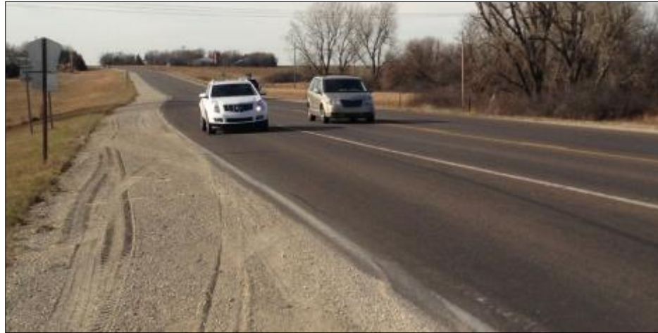
Figure 4.1 Use of by-pass lane
