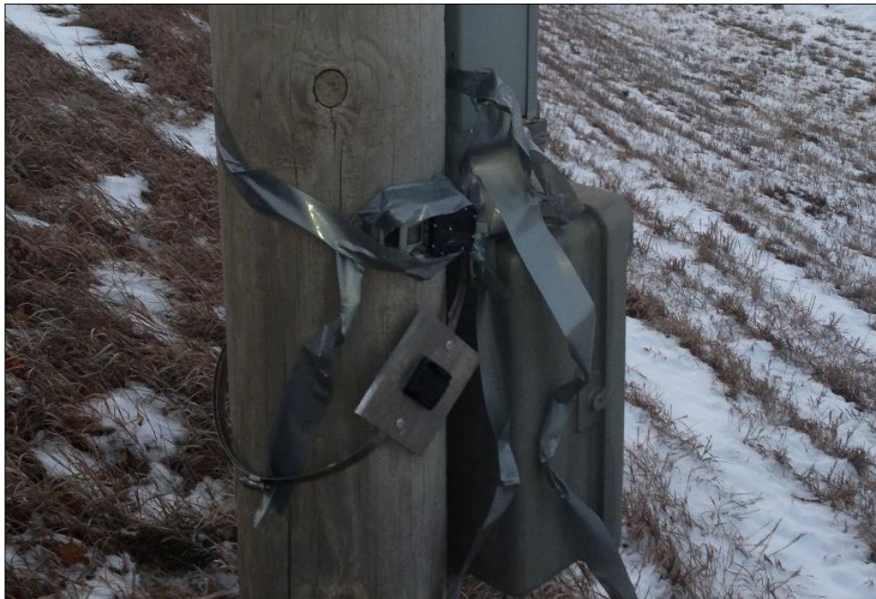
Figure 3.12 Installed Go-pro camera on pole
