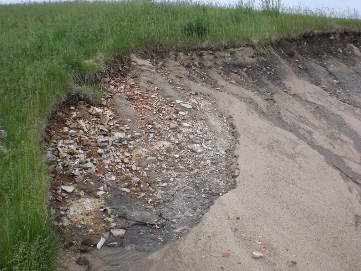
Figure 2.61 – Bunker Subgrade Material Contamination, Colbert Hills Golf Course, Manhattan, Kansas (Author)
