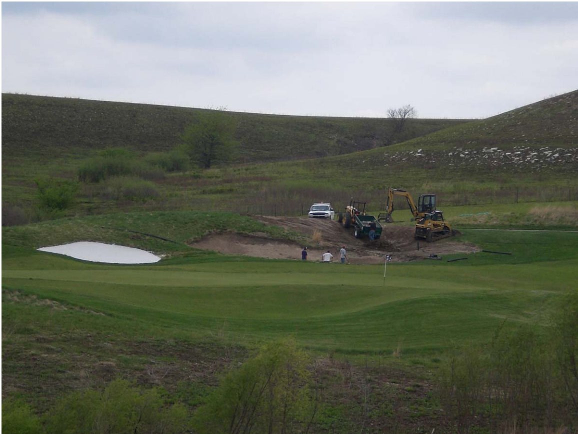
Figure 2.64 – Bunker Renovation Construction, Colbert Hills Golf Course, Manhattan, Kansas (Author)
