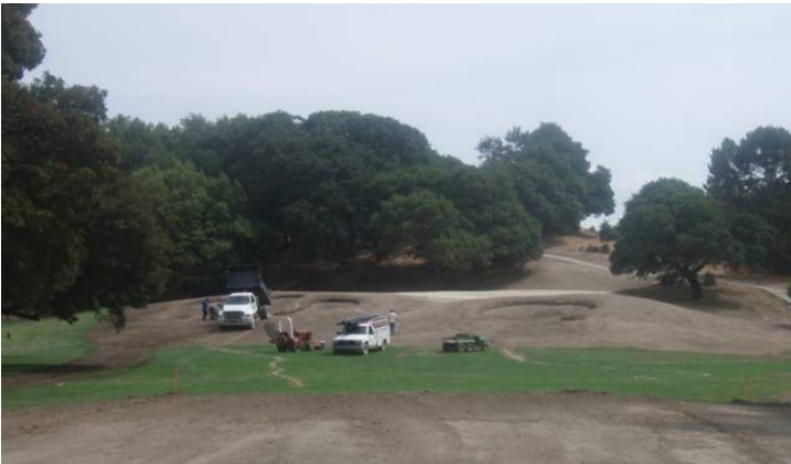
Figure 2.66 – 3 rd Hole Peacock Gap Golf Club During Construction (Forrest Richardson & Associates)
