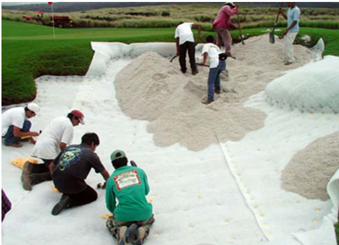
Figure 2.37 – Installation of Bunker Liner and Sand (sandmat.com)
