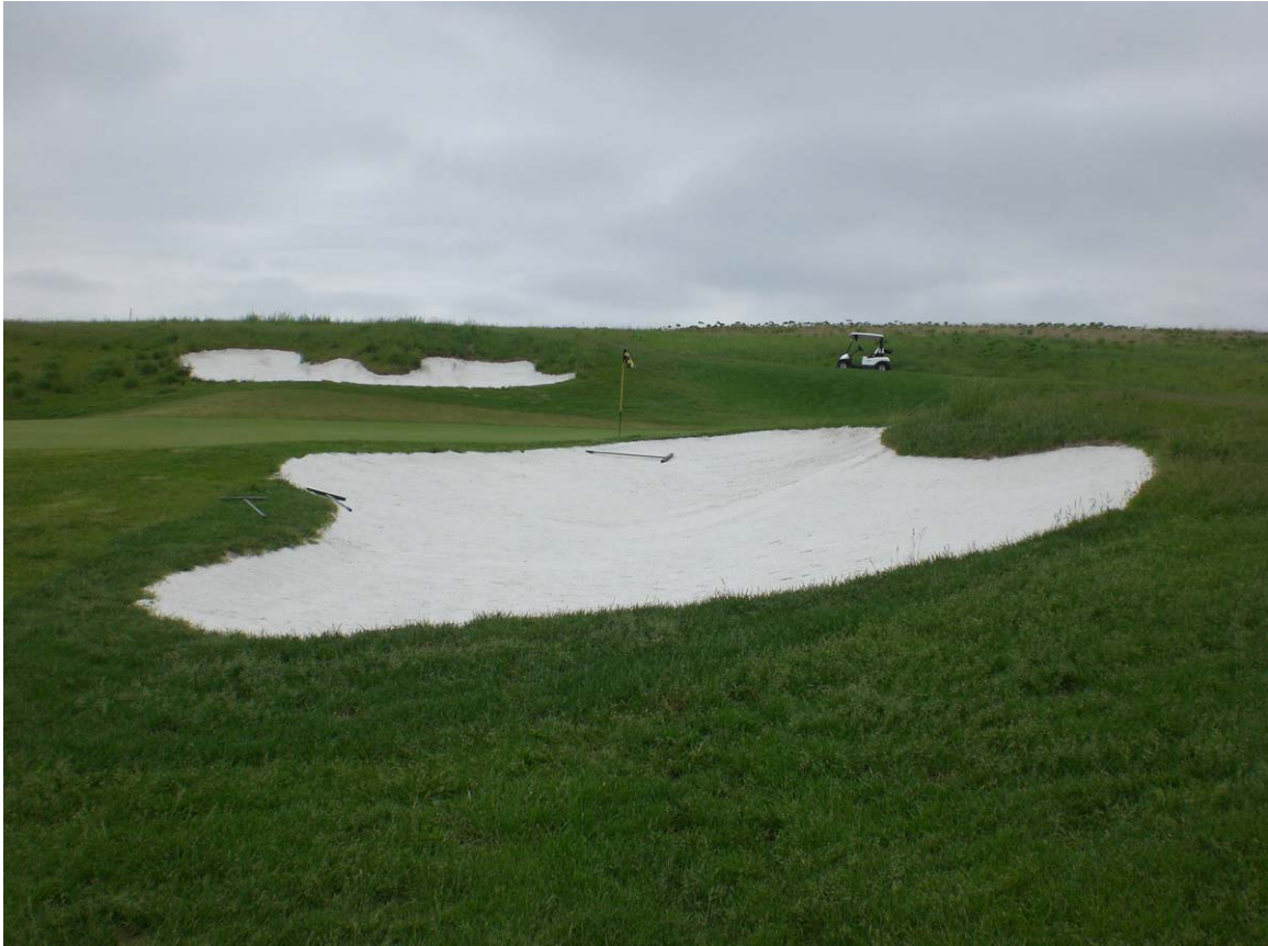
Figure 2.62 – Renovated Bunkers, Colbert Hills Golf Course, Manhattan, Kansas (Author) – This image was taken following the same rain event that caused the significant damage seen in Figures 2.59 – 2.61)
