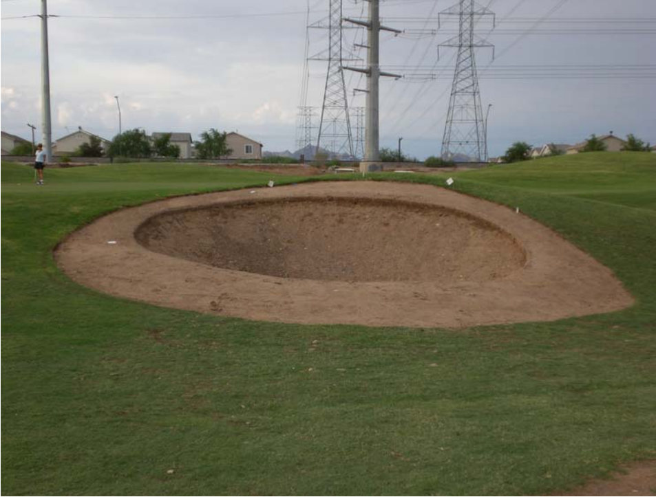
Figure 2.35 – Bunker Following Final Shaping, Hole 2 Coldwater Golf Course, Avondale, Arizona (Author)
