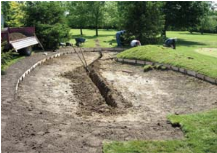
Figure 2.47 – Plywood Used for Bunker Edge Stability (clubandresortbusiness.com)
