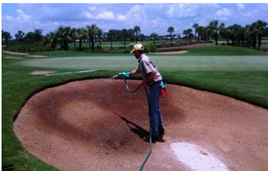
Figure 2.38 – Spray-on Liner Application (klingson.com)
