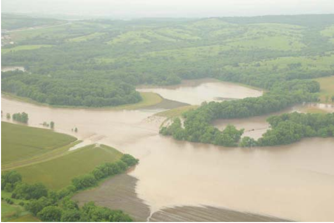
Figure 1.2 Aerial photo of 2011 flooding along Wildcat Creek at the project site (Photo by Rob Ott, City Engineer, 2011)
