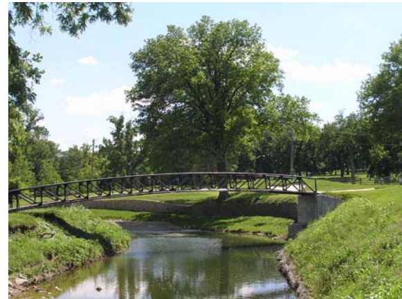
Figure 2.34 Bridge to hole seventeen green (Photo by author, 2012)
