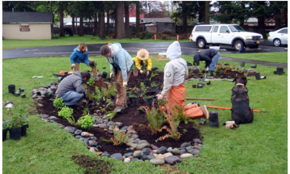
Figure 3.43: Rain garden being constructed on a property. (The City of Gresham, Oregon, 2012)
