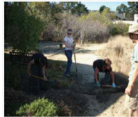
Figure 2.6: Trench connecting the upper and lower rain gardens
