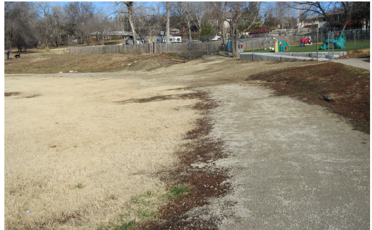
Figure 3.5 Current condition of track (author 2012).
