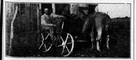
THIS tool can be made on the farm by any farmer or farm boy. Its chief use is as a hay cart, made by using an axle and two wheels of an old mower. The simplicity of this tool makes it light and above all, the safety hook on this cart is the outstanding feature.
