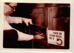
Question used in booklet for Method II. 28. Turn on \_\_\_\_\_\_ No. 2. Answer to question No. 27. off Slide No. 29. Picture of subject in position to turn off No. 2 fill valve. Circle arrow showing direction valve should be turned.
