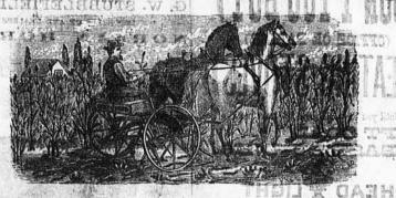
Experience has proved that Knives Spirally arranged on a cylinder cut stalks better than streight knives. The draft is much lighter, and the AVERY is the most durable cutter made. Inquire for the Avery, don't be put off with any other. If your dealer does not keep it, send to us for full particulars.
