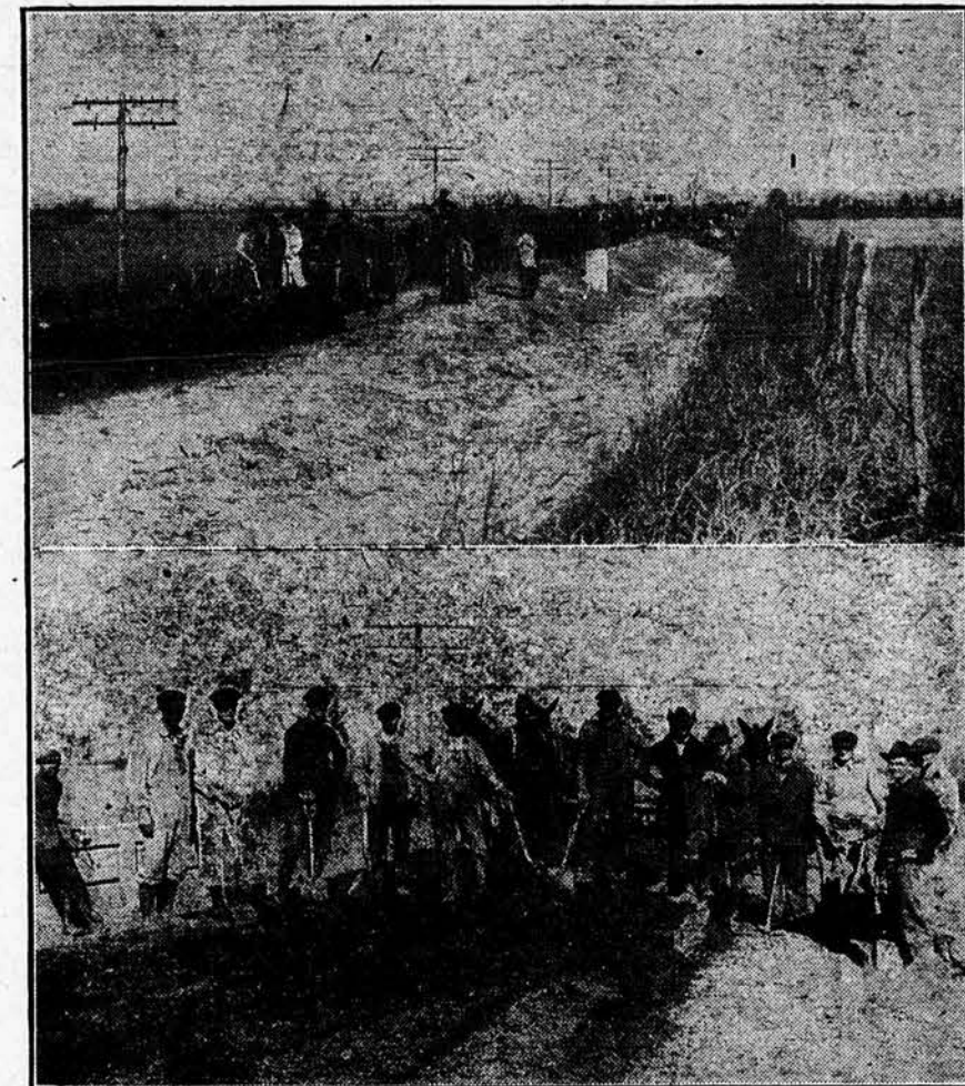
Above—Farmers and Teams Hauling Gravel for the New Road in Labette County. Below—A Few of the Road Builders Placing Gravel.
