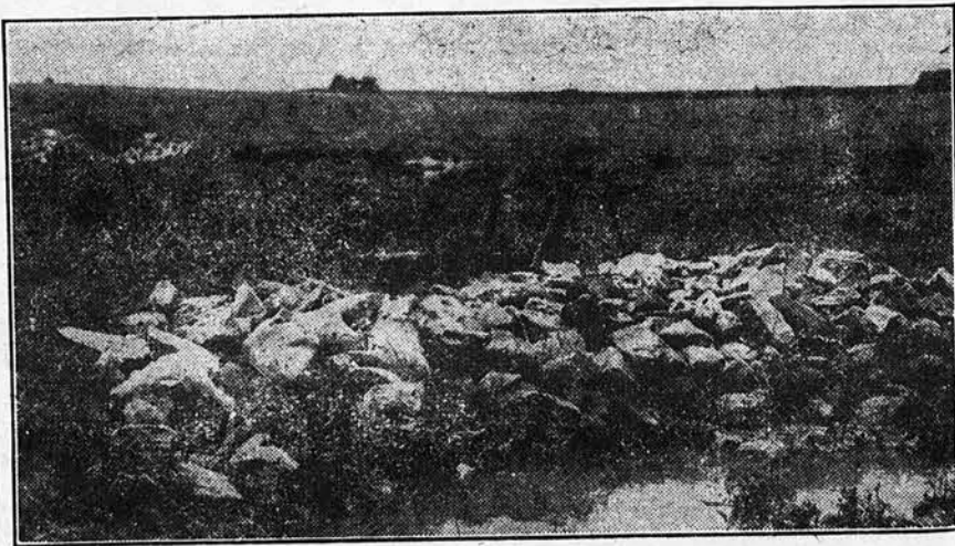
These Loose Rocks Were Gathered From the Fields and Are Now Serving Better Ends in Saving a Gully From Washing
