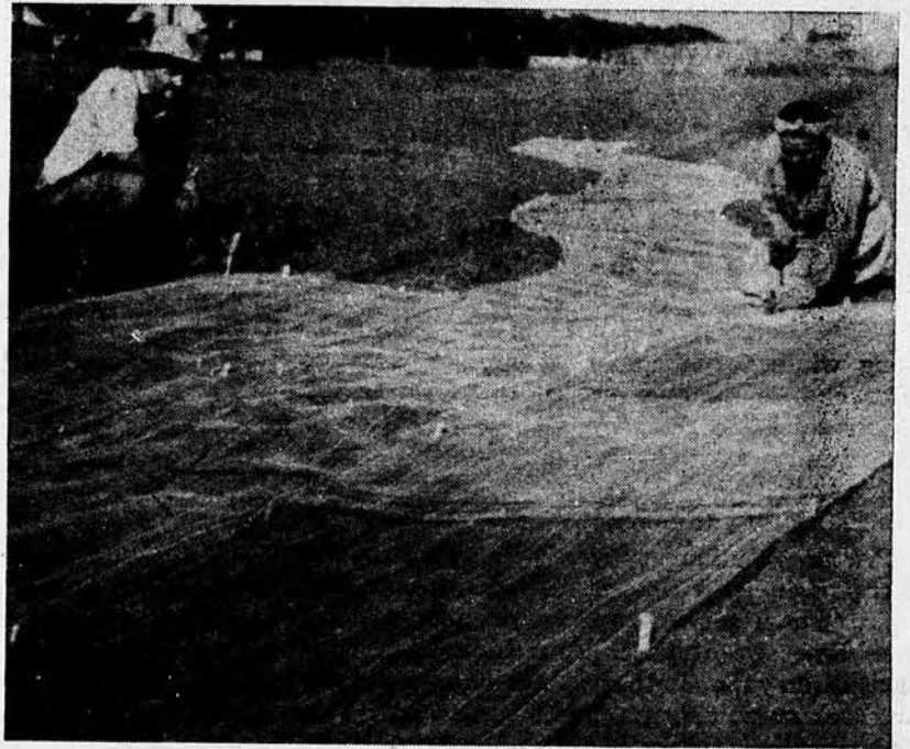
Willis Colman and his daughter, Waneta, shown pegging down soil erosion control netting in waterways on their farm in Douglas county. These waterways had been filled in and widened with a slip, then seeded to brome grass. This picture was taken August 19, 1946.
