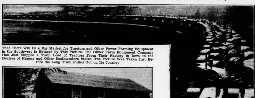
Interesting Farm Home of N. B. Swink, Seward County. It Has Full Concrete Basement But the Walls Are Adobe, Made From the Soil Taken From the Basement Excavation and Mixed With Wheat Straw. It Required 2,400 Such Bricks Made at a Cost of \$70 a Thousand. Stucco Finish and Porches Are to Be Added Next Spring. The Main Floor Has Five Rooms and Bath, and the Basement Four
