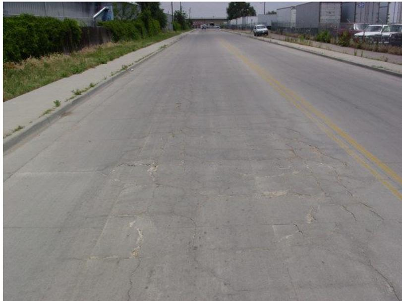
**Figure 2.11 Stop Sign Approach Distressed Area Observed at Santa Fe Drive Site (Sheehan et al., 2004)**
