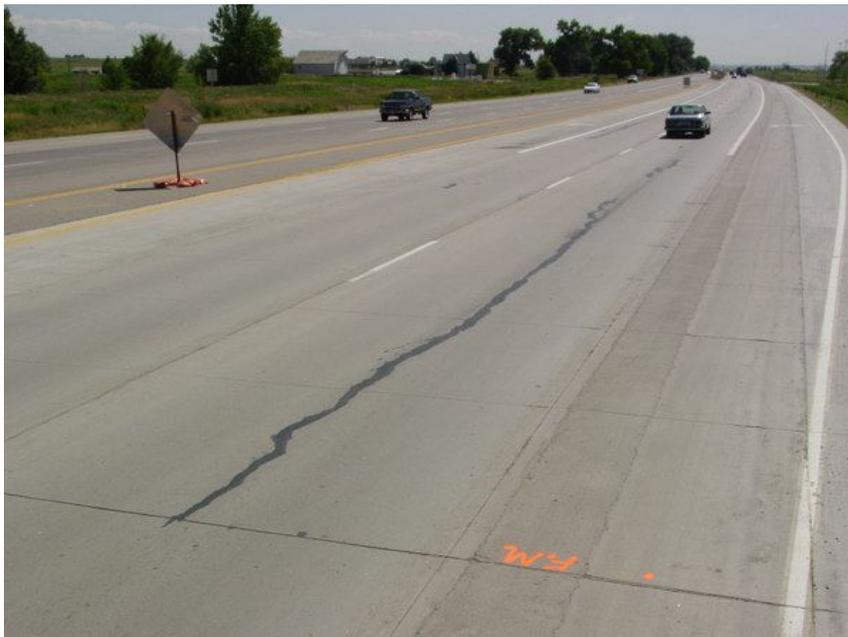
**Figure 2.13 Typical Slab Cracking Observed in S.H. 119 Test Section No. 2 (Sheehan
