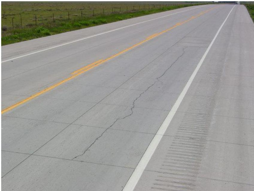
**Figure 2.15 Typical Cracked Slab Conditions Observed at the U.S. 287 Lamar Site (Sheehan et al., 2004)**
