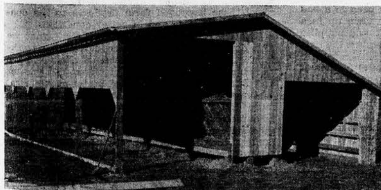
This practical feeding and loafing barn, also designed by Ernest Harms, will house and feed 100 cows at a time. It is 25 by 50 feet in dimensions.
