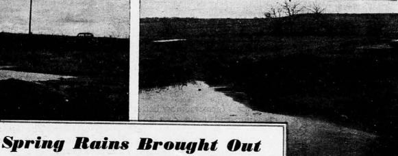
Foreign drainage from across the road broke thru a dike and tore up this terrace in Coffey county. Terrace fills across depressions of this kind should be at least 6 inches higher than on either side.
