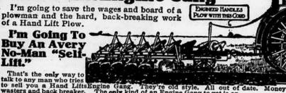
The Plow that handles itself. A special Automatic "Power Lift-Self Drop" Device takes the place of the usual hand levers. No plowman is needed. Saves you all the expense of his wages and board. One man runs both the engine and the plows. At the ands of the furrows all he has to do is to pull a cord to engage a clutch and the plows are automatically raised or lowered. No hard back-breaking work lifting and lowering the plows by hand levers. The "Power Lift-Self Drop" Device does all the work.
