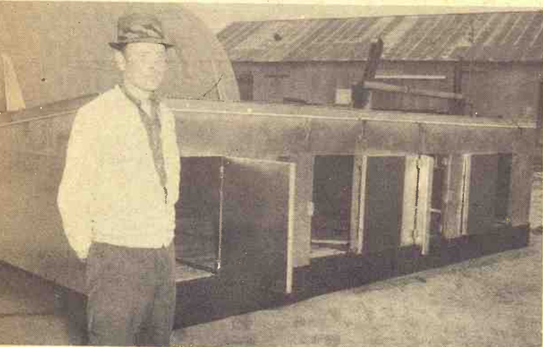
The new design of farrowing houses is shown in this view with John Lamoreaux. Doors are hinged to swing out and up for best ventilation. All buildings are insulated, farrowing houses and nurseries equipped with heat lamps. Operators believe this type of equipment lends itself to a near disease-free operation. Pigs receive both solid and liquid feeds.
