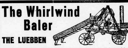
The ONLY Baler which will bale ALFALFA taken direct from the windrow and keep the ALFALFA in perfect condition, free from mold. A HOLE runs through the center of the bale permitting air to circulate and thereby curing the alfalfa. If you have Two Hundred Tons of Alfalfa this year, by baling it with the Luebben you will save the price of the Baler. Write us and we will show you
