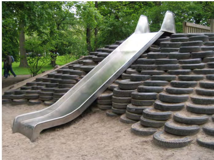
Figure 3.2.14: Tire Slide Earth filled tires are used to construct playground equipment in Leipzig, Germany. (Belanger 2010)
