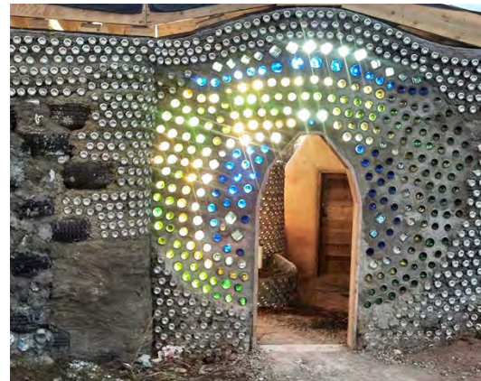
Figure 3.2.15: Recycled Walls Earthship structures in New Mexico are built of cans, bottles, tires, and concrete. (Parkins 2015)
