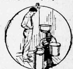
The constant speed of the electric motor means better separation of the cream.
